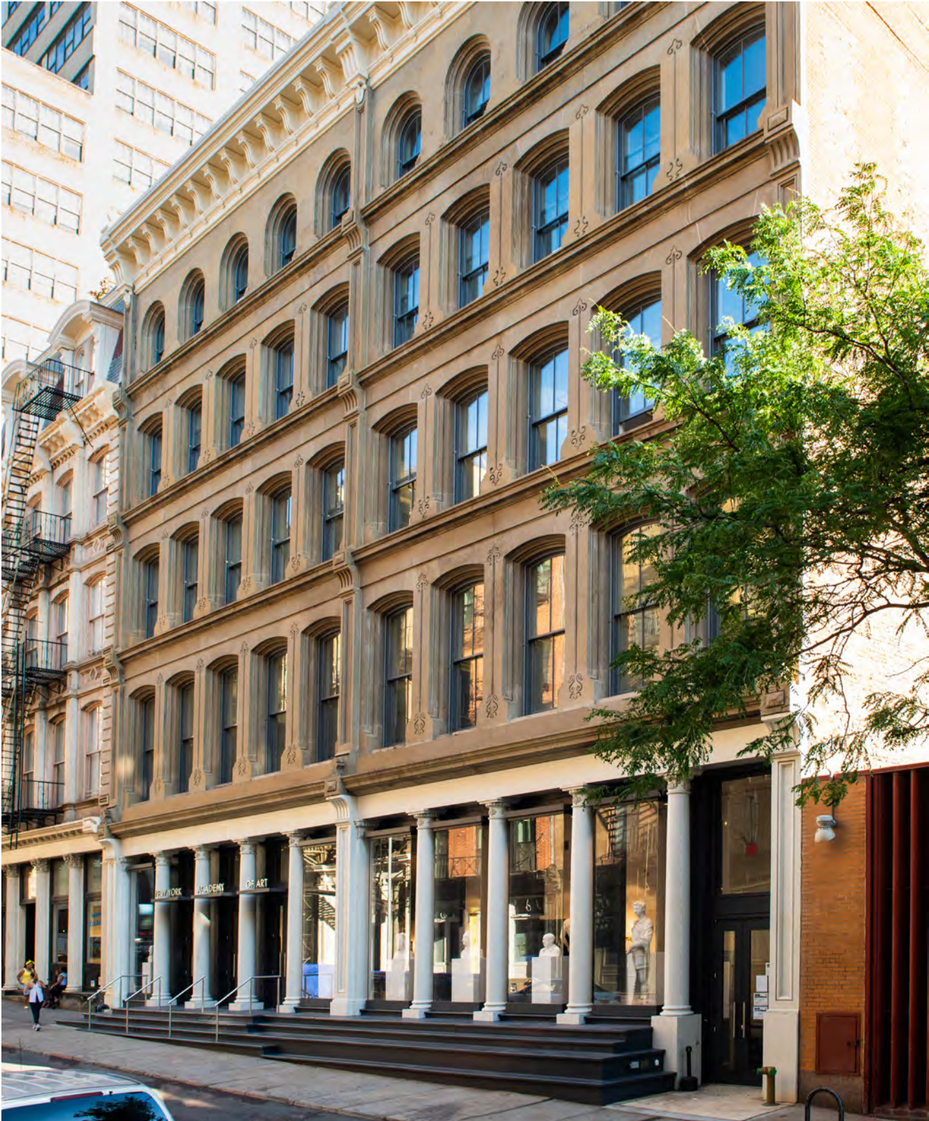
The Facade after the 2019 Restoration
