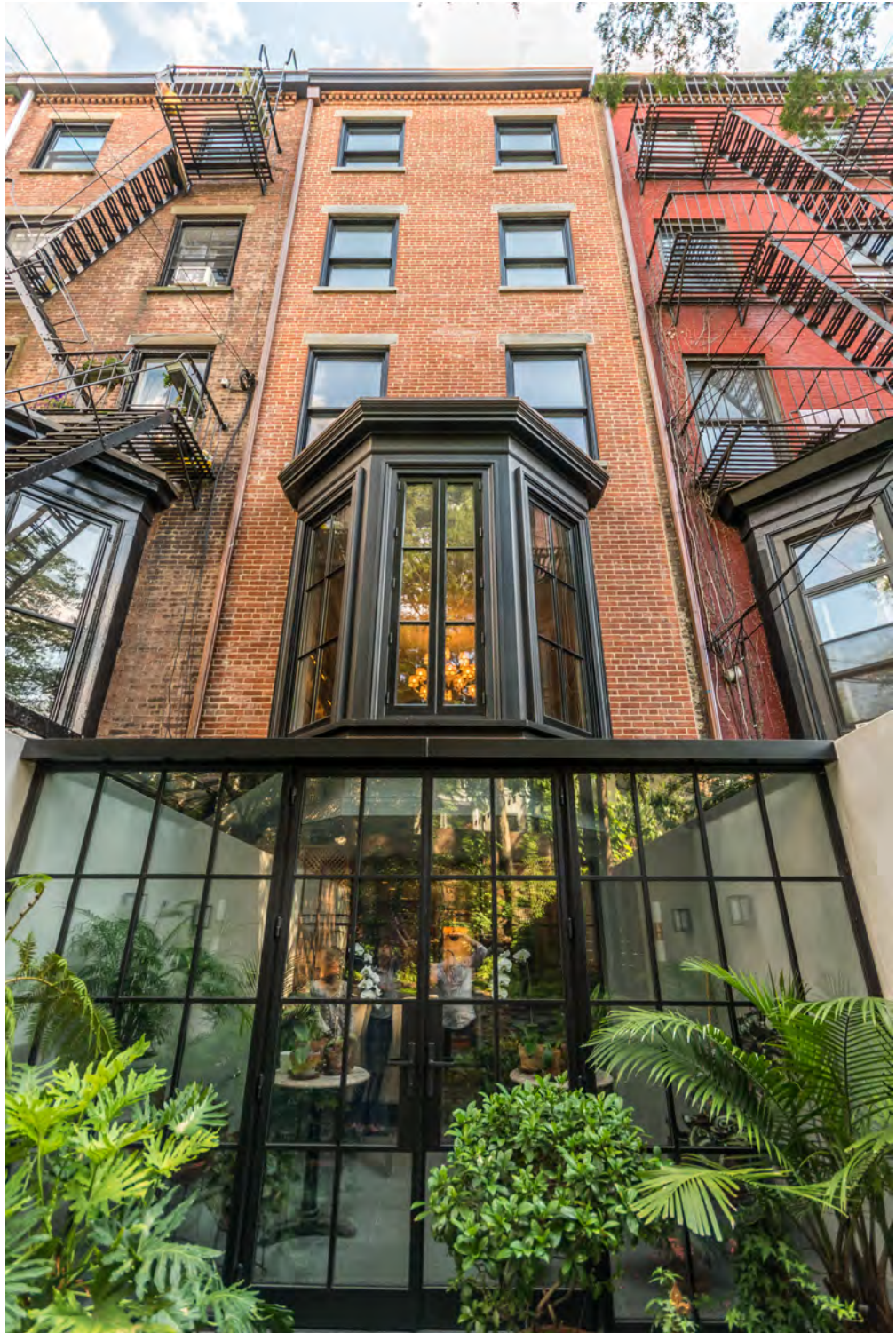
Rear Facade after the Restoration: view of the new Conservatory
